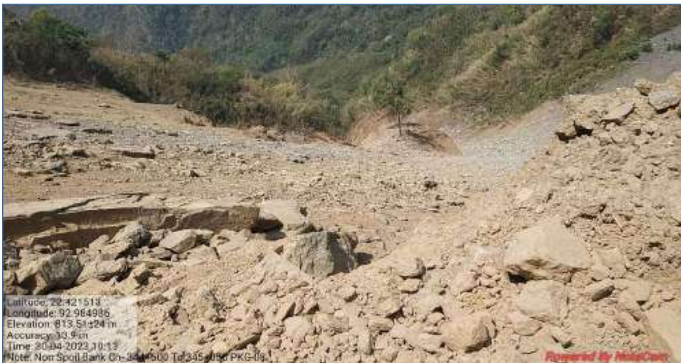
Additional Spoil Bank-1 km-344+825 (Bottom Level Surface)
