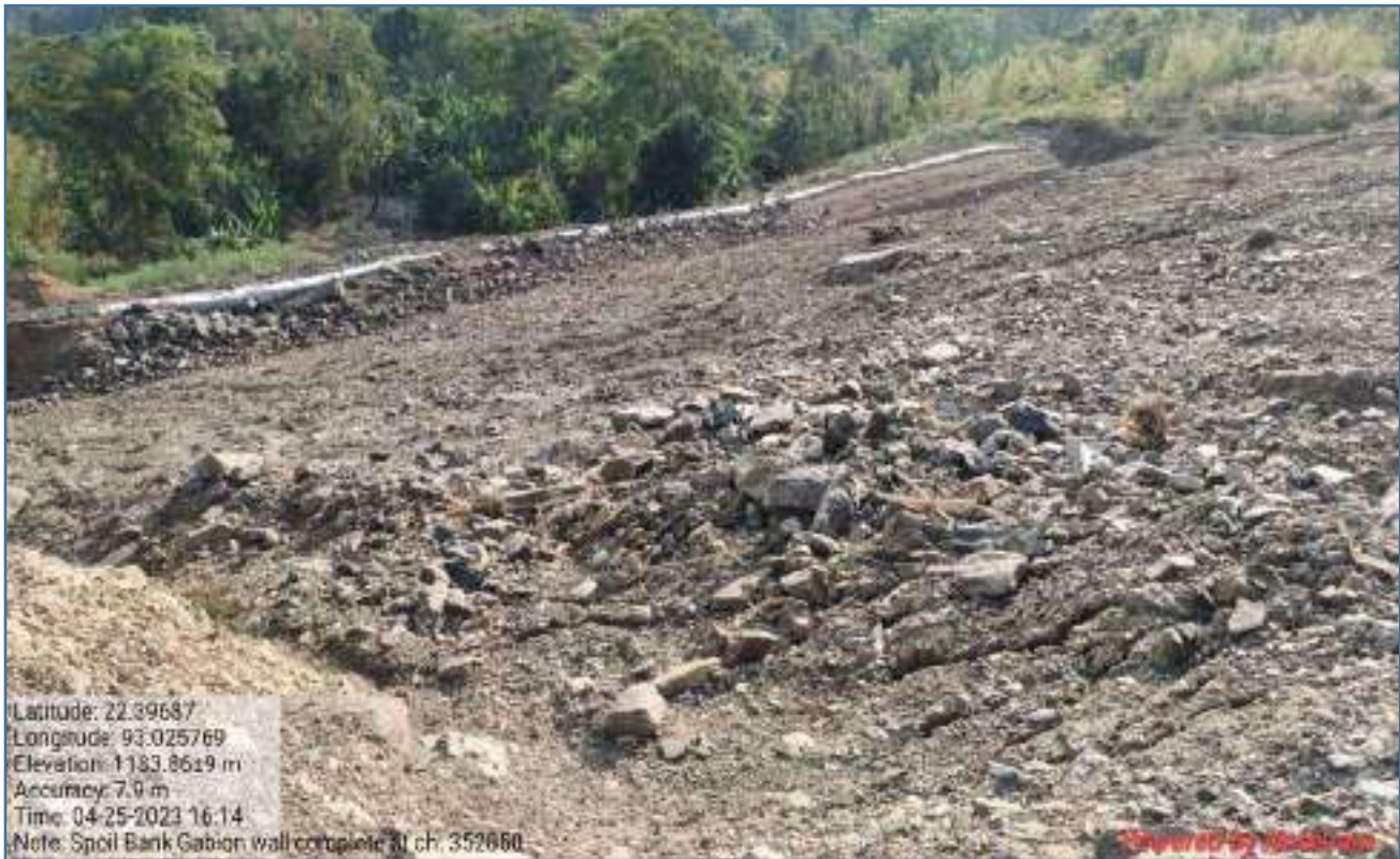
Spoil Bank- 8 km 352+840 (Bottom Level Surface)
