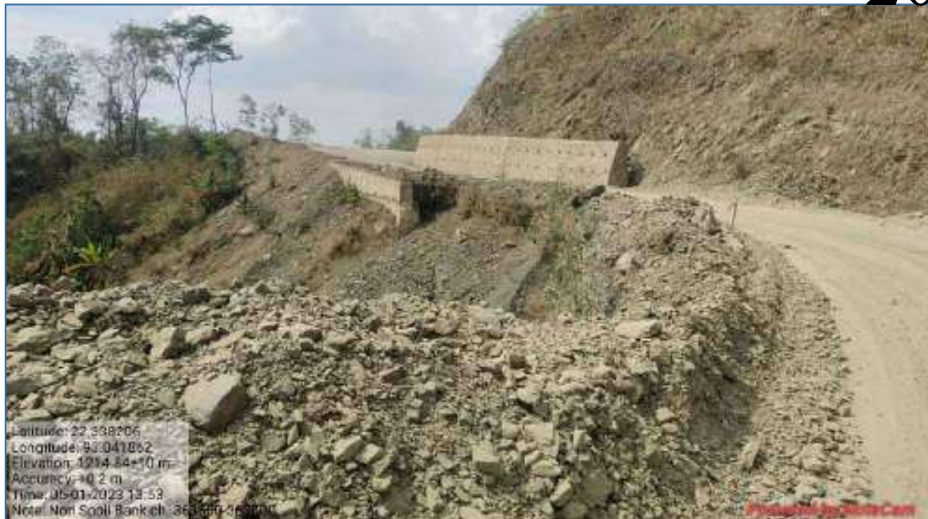
Additional Spoil Bank - 5 km-363+700 (Road Level Surface)
