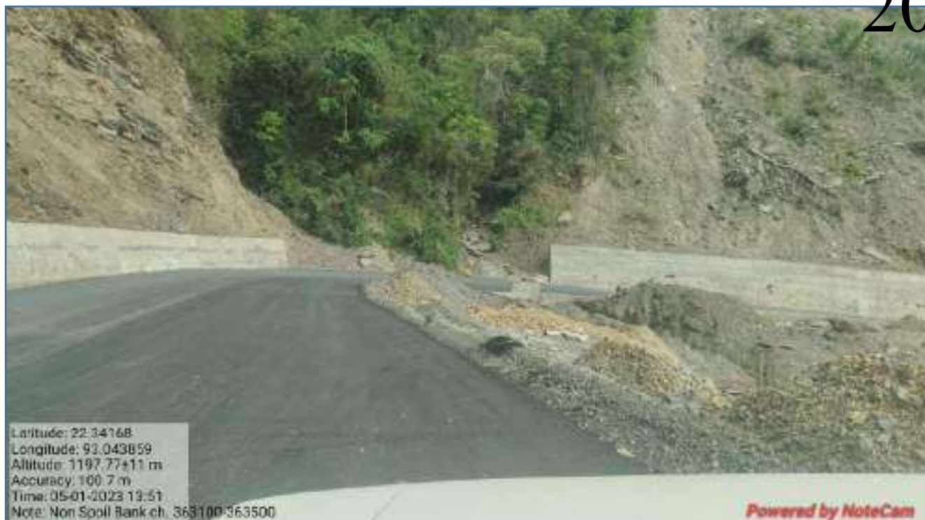
Additional Spoil Bank -4 km- 363+300 (Road Level Surface)
