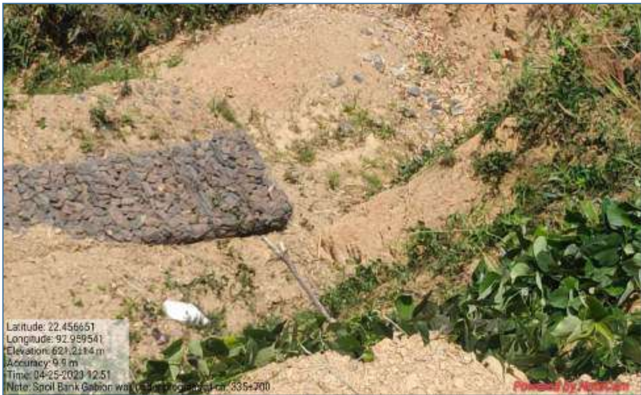
Spoil Bank-1 Km 335+655 (Bottom Level Surface)
