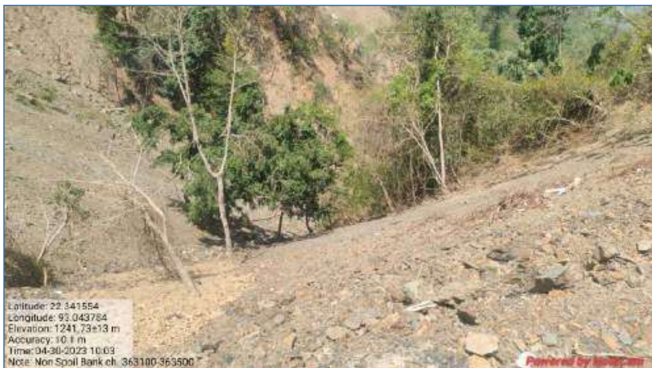
Additional Spoil Bank -4 km- 363+300 (Bottom Level Surface)
