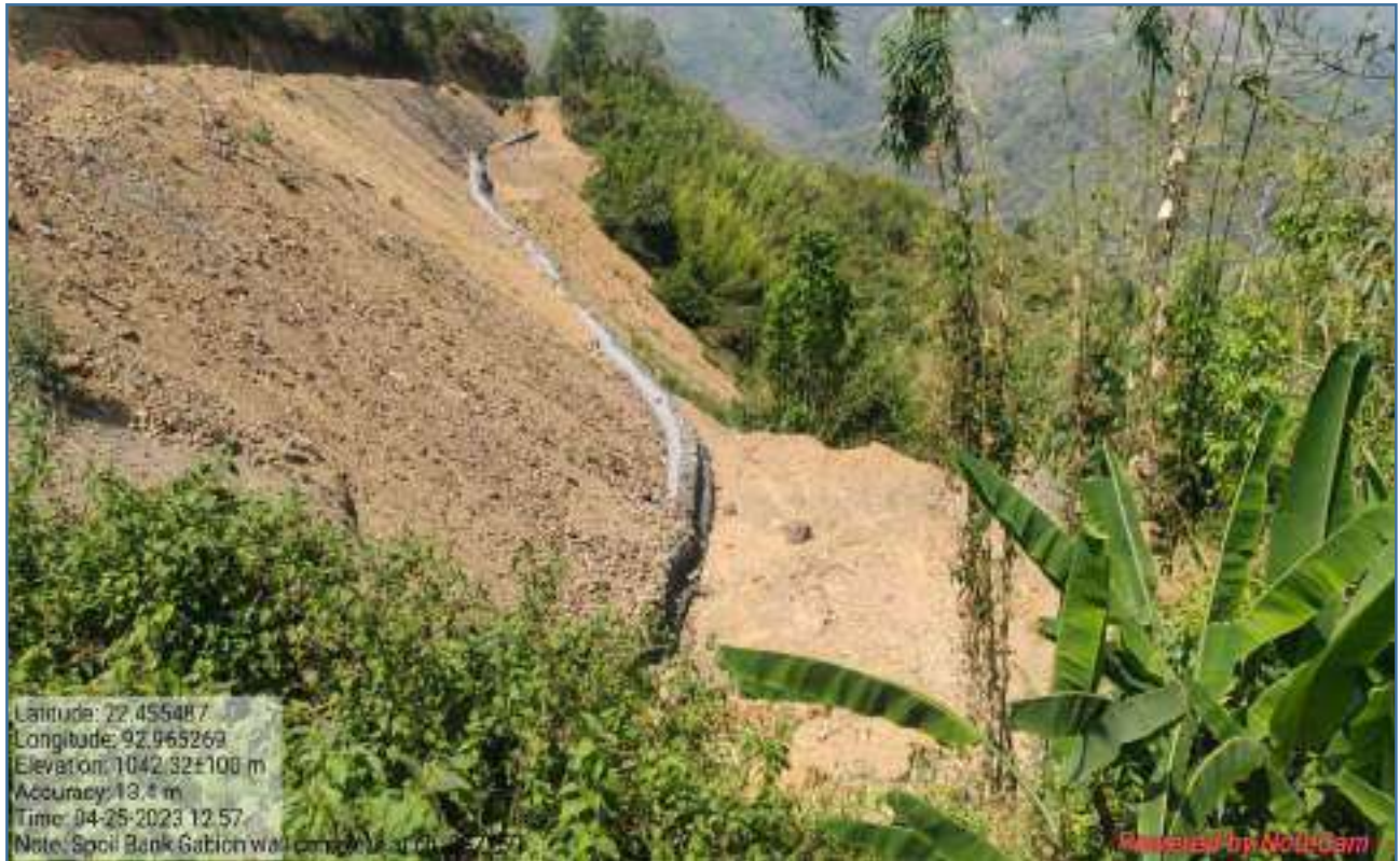
Spoil Bank- 3 km 337+180 (Bottom Level Surface)
