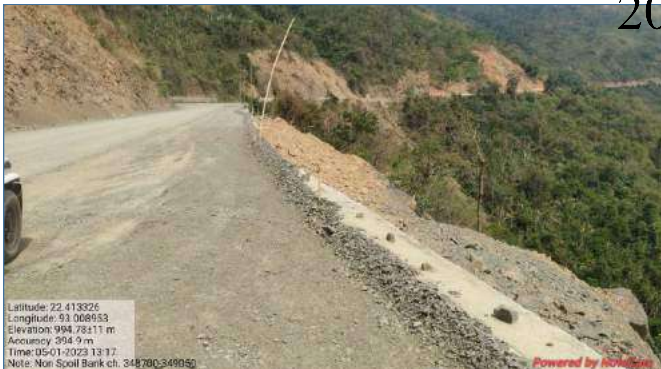
Additional Spoil Bank-2 km-348+875 (Road Level Surface)
