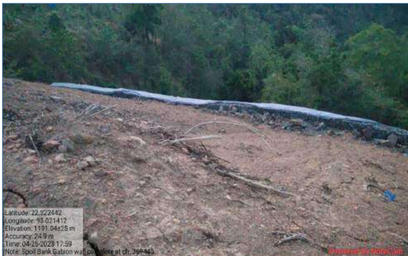
Spoil Bank-13 km – 369+440 (Bottom Level Surface)
