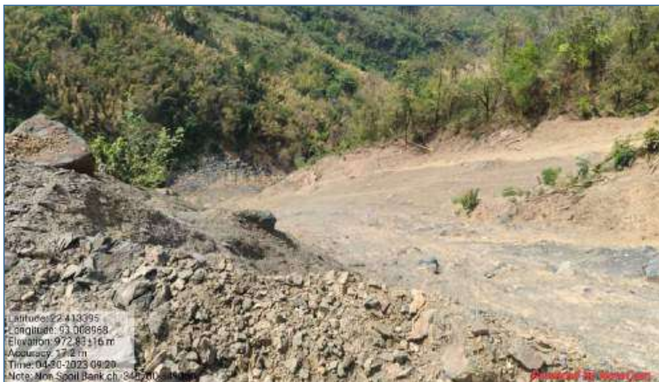
Additional Spoil Bank-2 km-348+875 (Bottom Level Surface)
