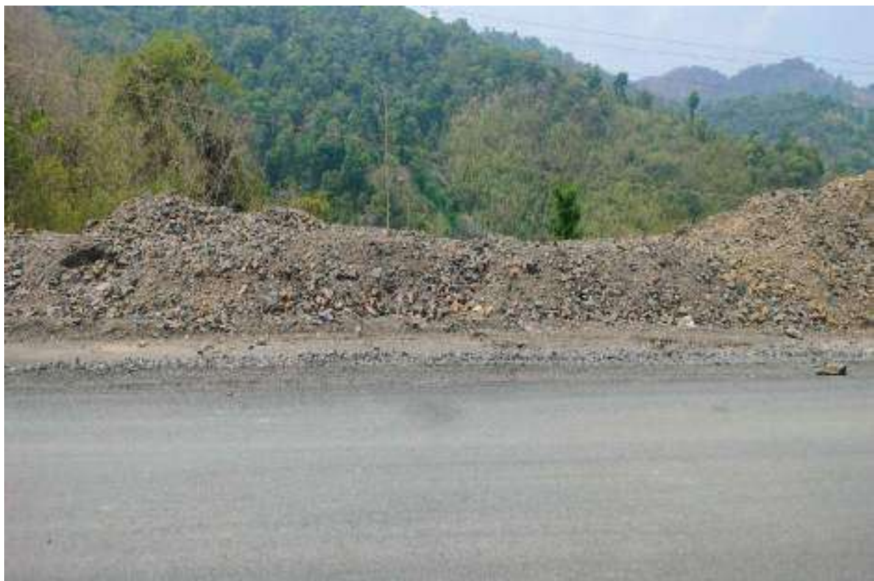
Additional Spoil Bank – 300+960 to 301+010
