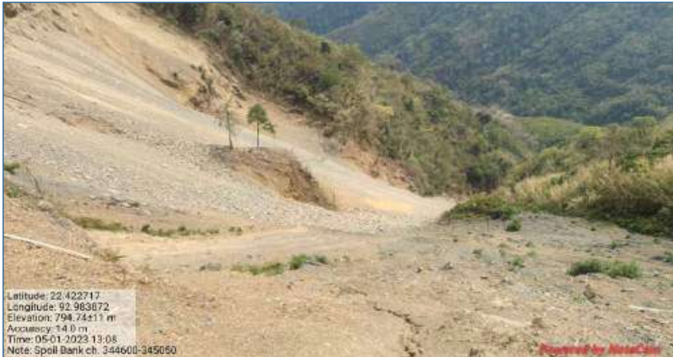
Additional Spoil Bank-1 km-344+825 (Road Level Surface)
