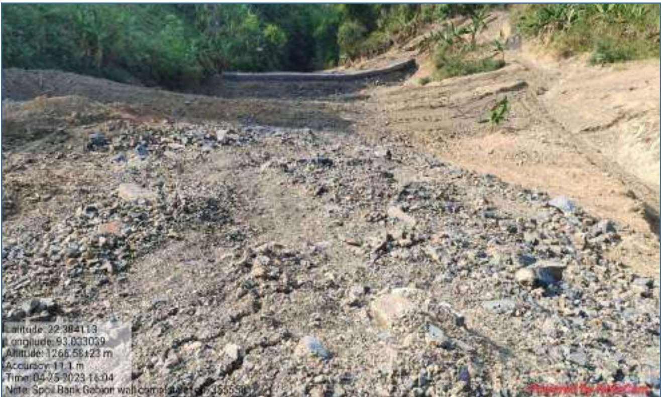
Spoil Bank-11 km 355+552 (Bottom Level Surface)
