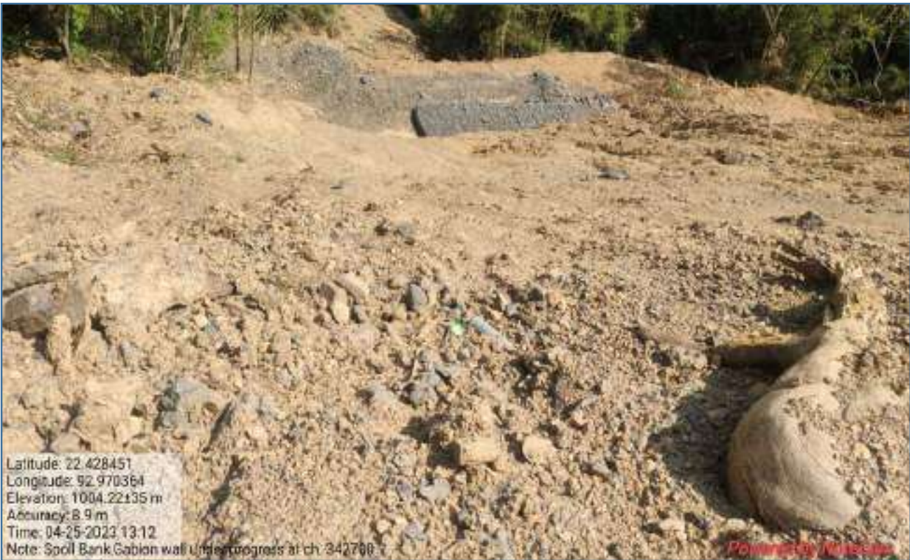
Spoil Bank- 7 km 342+700 (Bottom Level Surface)
