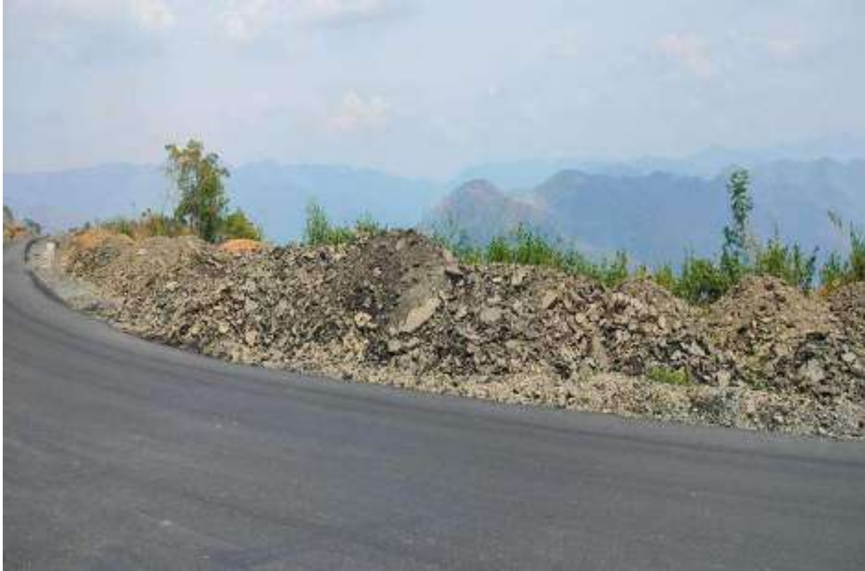
Additional Spoil Bank – 307+220 to 307+280
