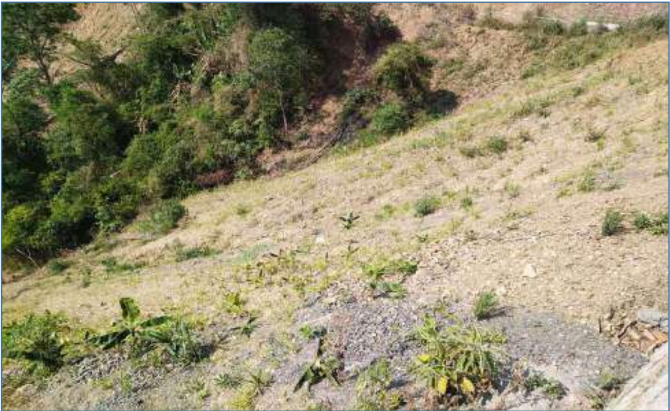
Spoil Bank-10 km 354+450 (Bottom Level Surface)
