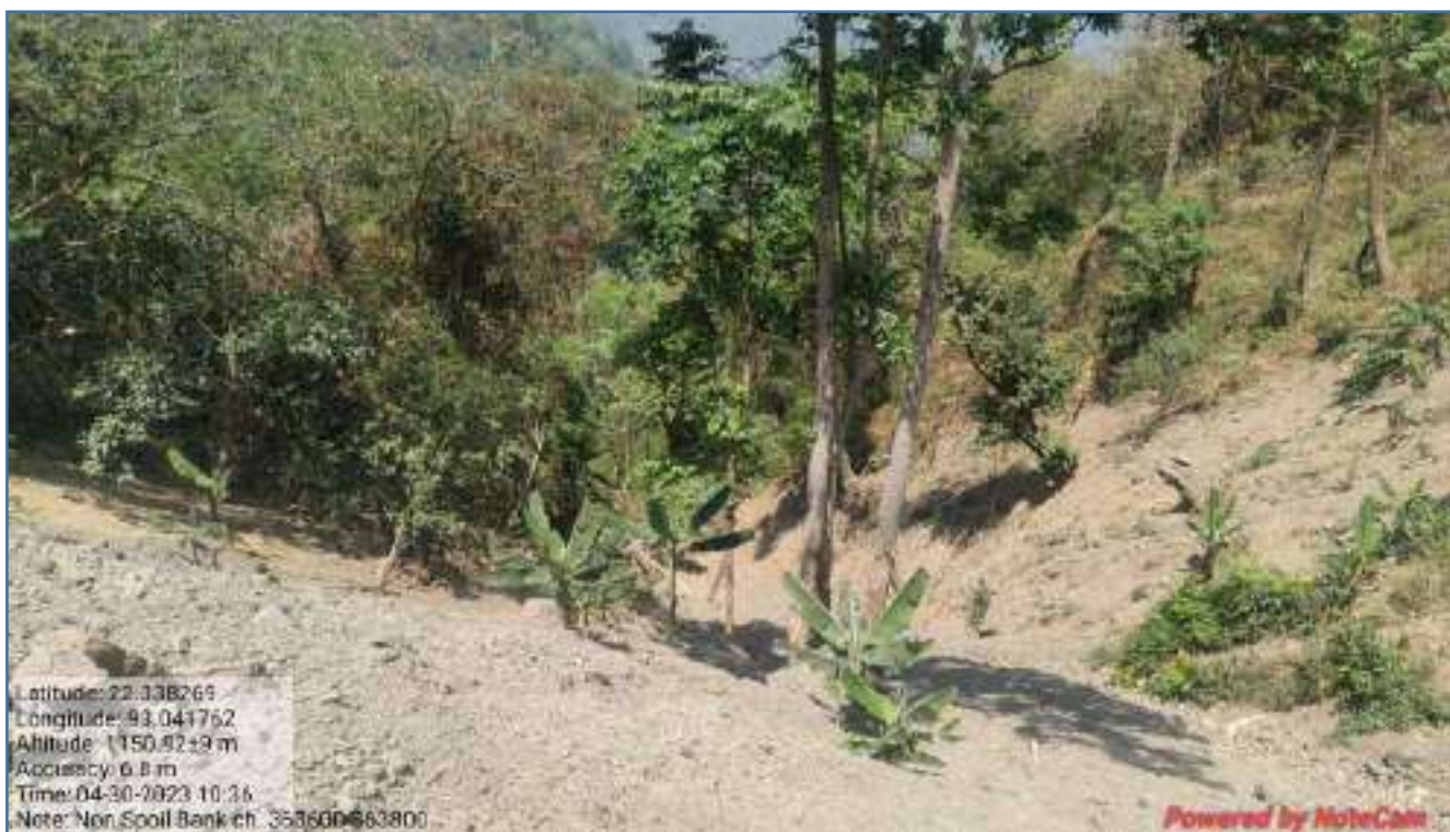
Additional Spoil Bank - 5 km-363+700 (Bottom Level Surface)
