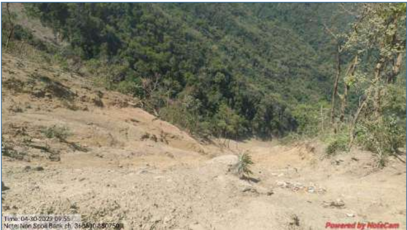
Additional Spoil Bank -3 - km-360+675 (Bottom Level Surface)
