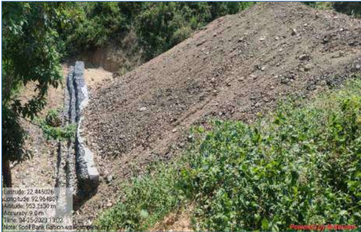
Spoil Bank- km 339+762 (Bottom Level Surface)
