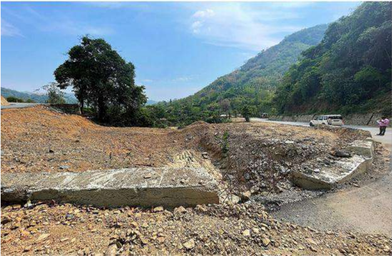
Additional Spoil Bank – 301+770 to 301+820
