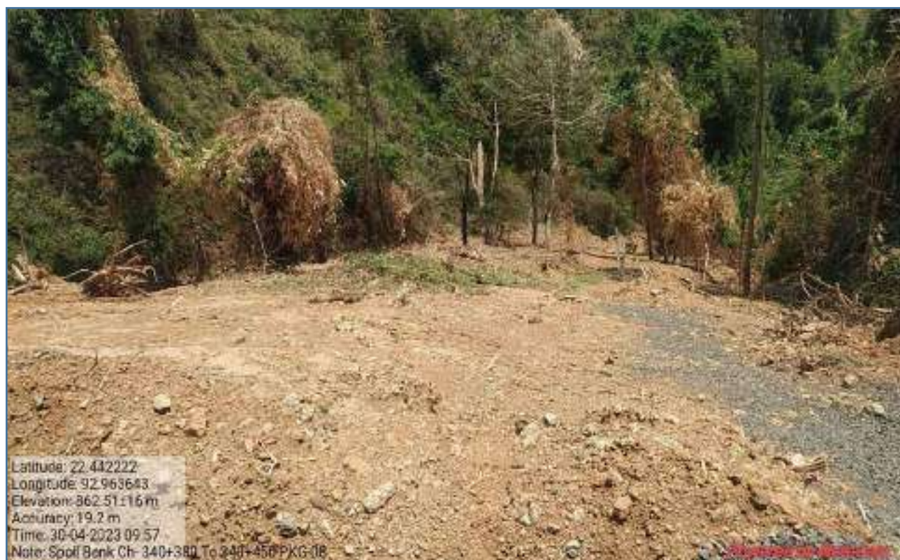
Spoil Bank-5 km 340+415 (Bottom Level Surface)
