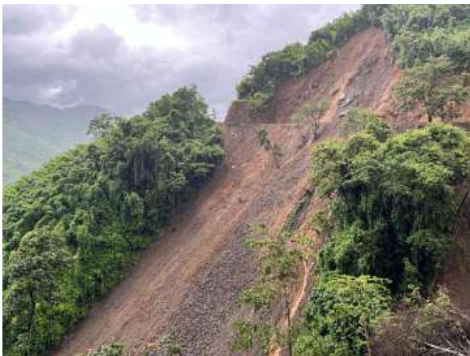
Photo showing muck sliding down the hill and damage to trees
