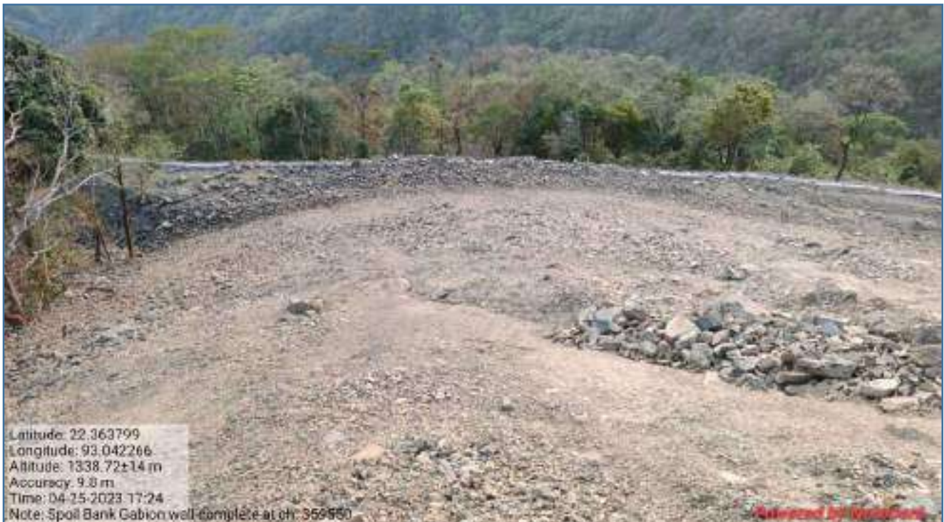
Spoil Bank-12 km 359+500 (Bottom Level Surface)
