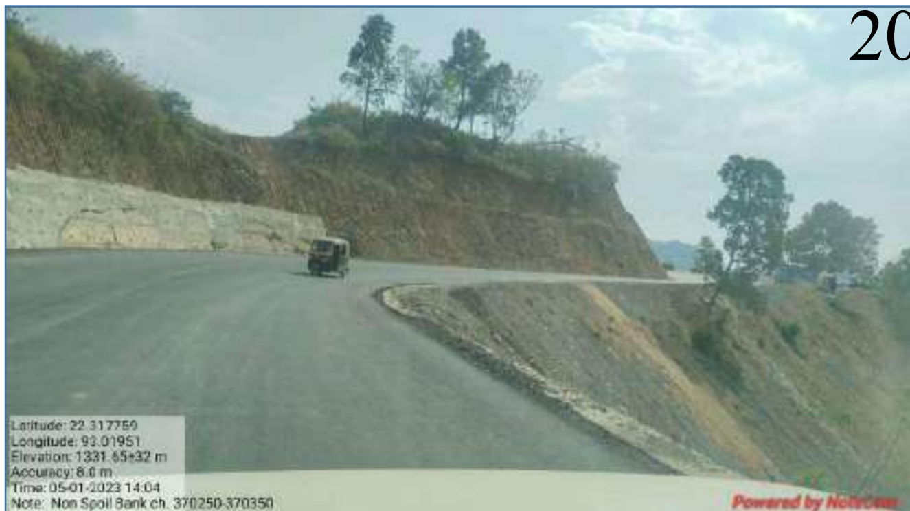
Additional Spoil Bank -6 Km – 370+300 (Road Level Surface)
